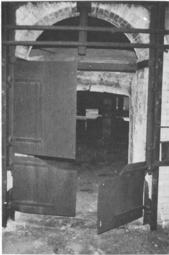
Close-up of one of the furnace doors. The pot would sit just inside. If you look closely, you can see the hole in the middle of the floor where the glass would go, if a pot broke.
