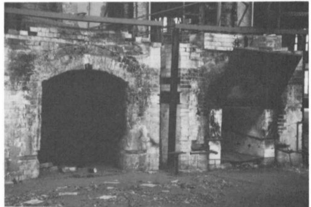
These small ovens were close to the furnaces and were used for warming the pots.
