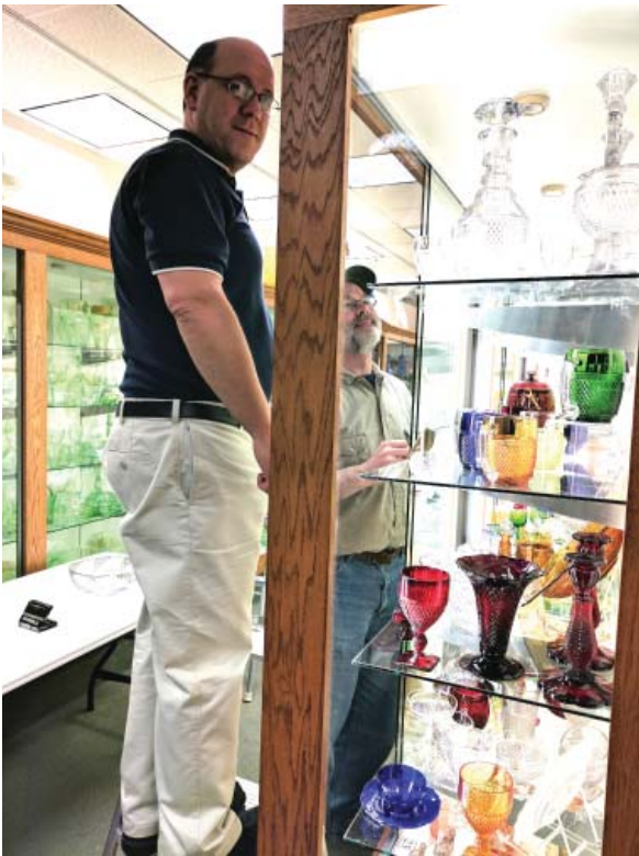
David Ray and Jack Thompson helped install the new LED light bulbs before the museum opened for the season.
