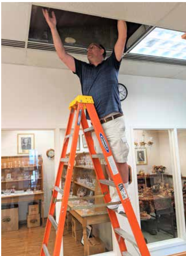
David Ray went up the ladder to change a few ceiling tiles. Thank you!
