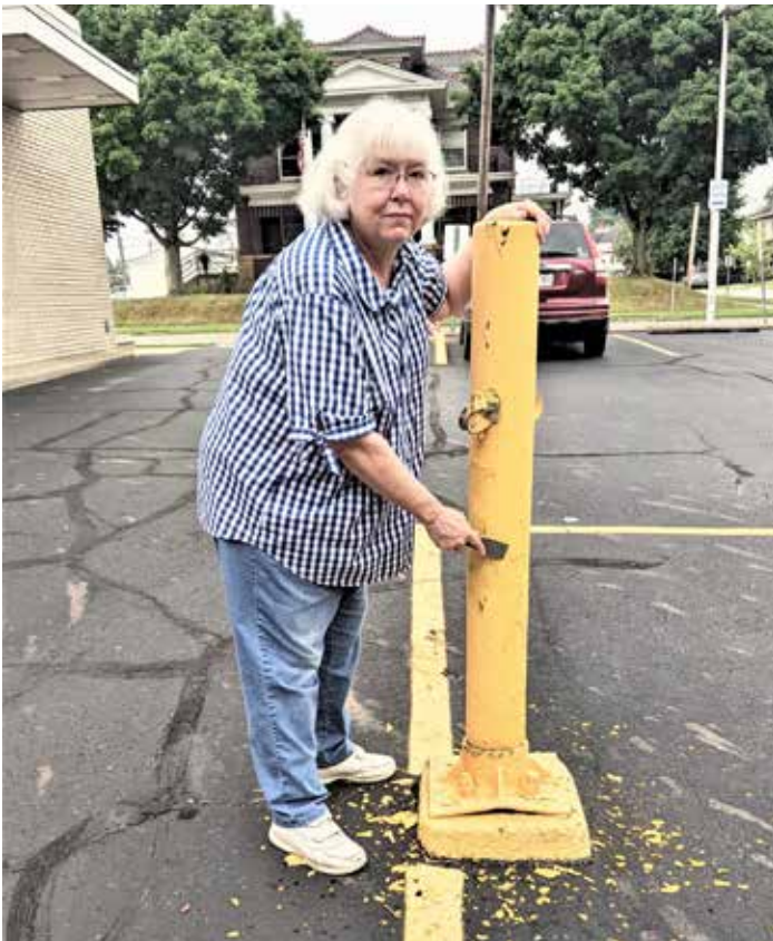
Before the Museum parking lot could be sealed and lined, volunteers scraped the loose paint from the curbs and pole. Lindy Thaxton is shown scraping off layers of paint.
